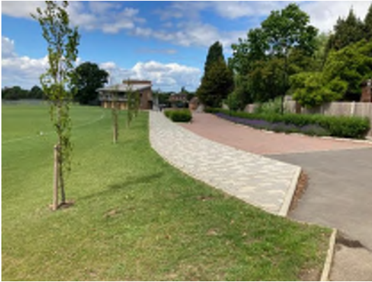
Wade side car park – looking towards pavilion
