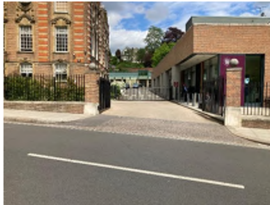
Main (South) entrance
