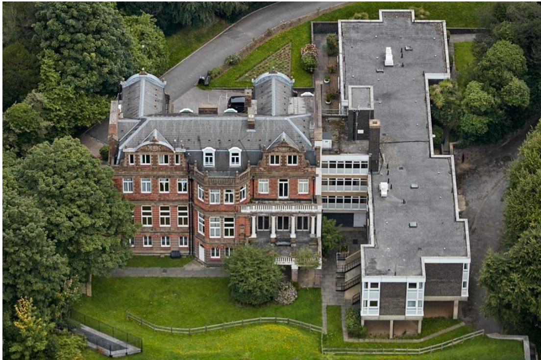
Figure 2.0 – Branch Hill Manor House (left) with abutting 1960s structure (right)
