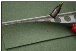
Plant E strips torch-bonded for bituminous systems
