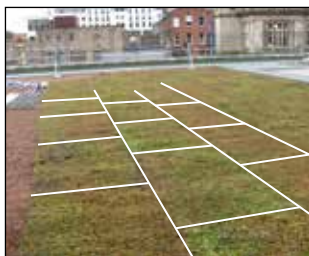
Lines indicate staggered brick pattern
