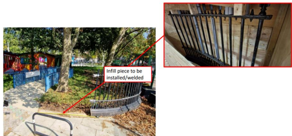
Figure 2. Location of missing railing (E/27) to be reinstated.
