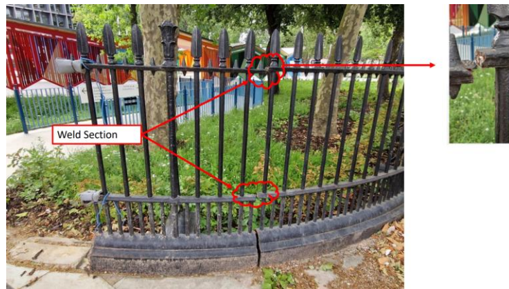
Figure 1. Panel E/28 showing locations for repair.
