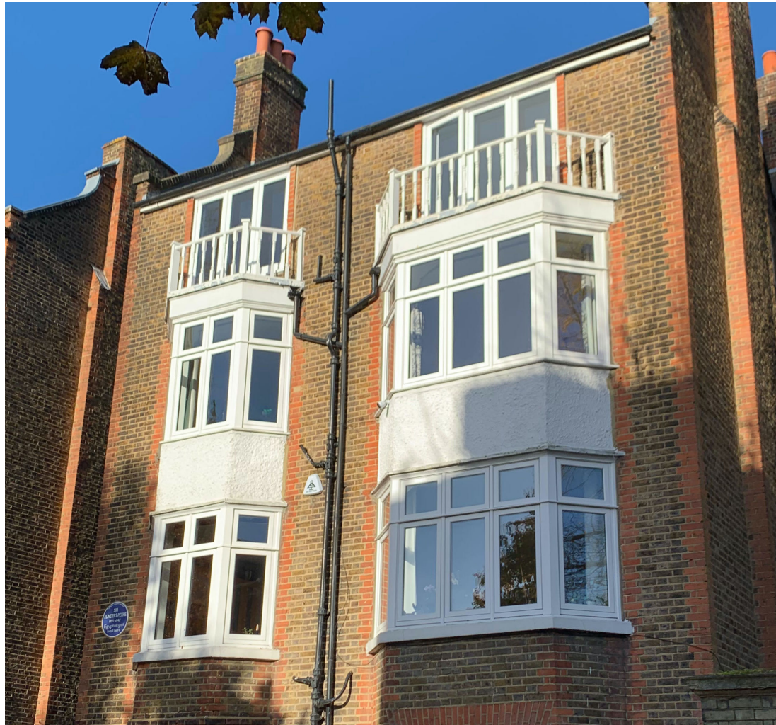
EXISTING WINDOWS ON SOUTH ELEVATION
