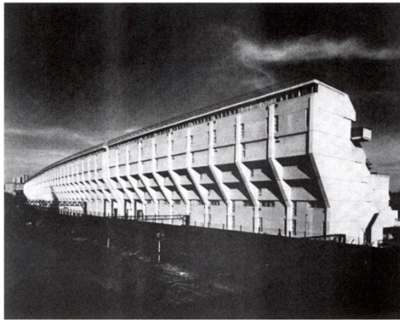
Rear Elevation Facing Train Line to the North
