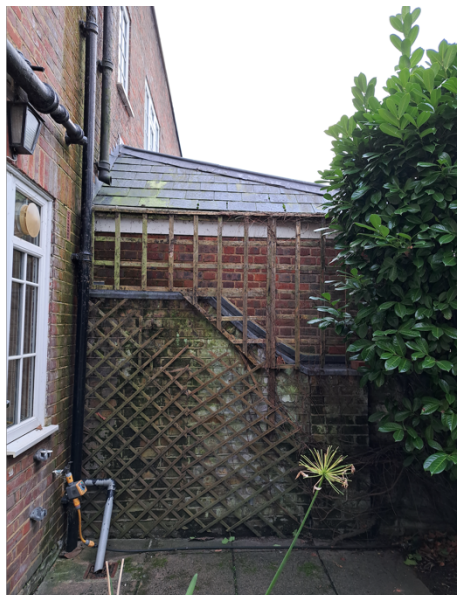
Figure 5: 8 Belsize Road extension
