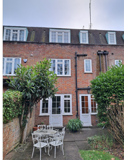
Figure 3: 6 Belsize Road, Rear elevation
