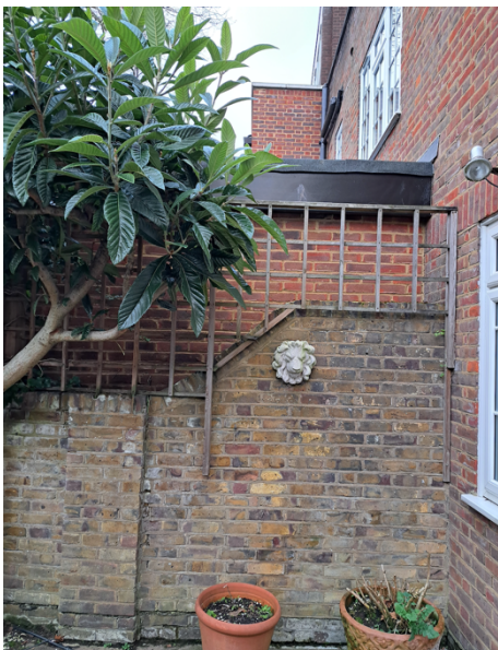
Figure 4: 4 Belsize Road extension
