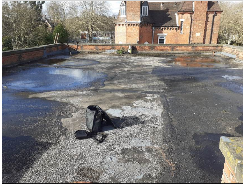
Fig 18 The uppermost flat roof to No 39a, showing the surrounding parapet
