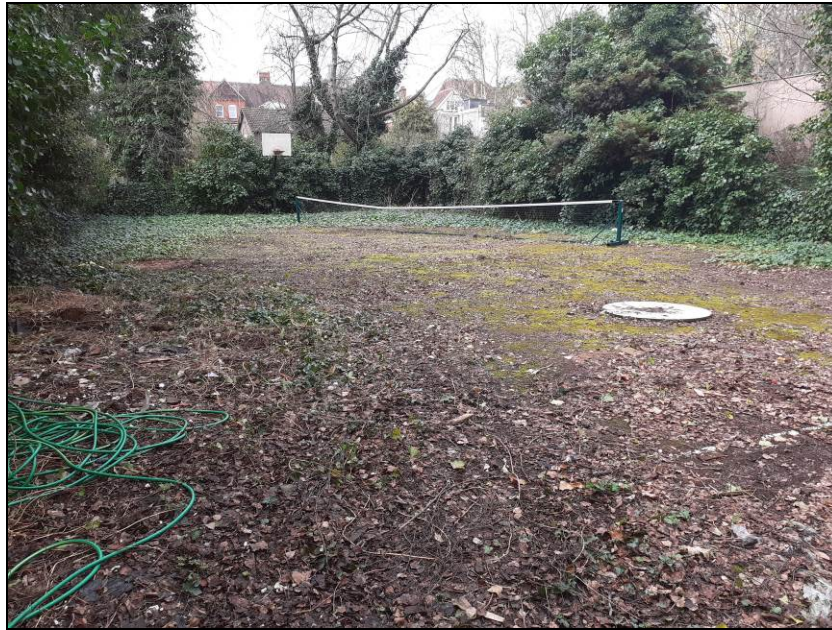
Fig 8 Derelict tennis court. Moss covering visible to the centre right of the photo, as is the encroachment of ivy at the margins
