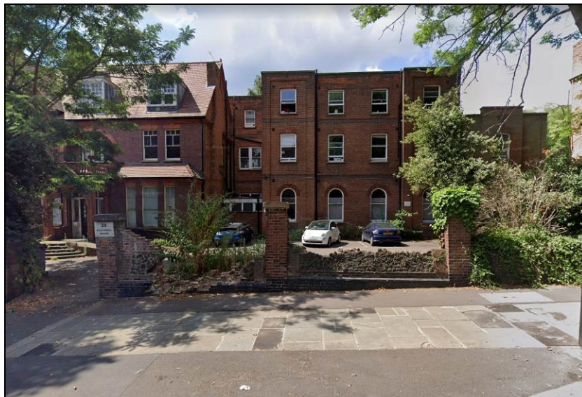
Fig 4 Front (east) elevation of 39a Fitzjohn's Avenue. No 39a is to the right.
