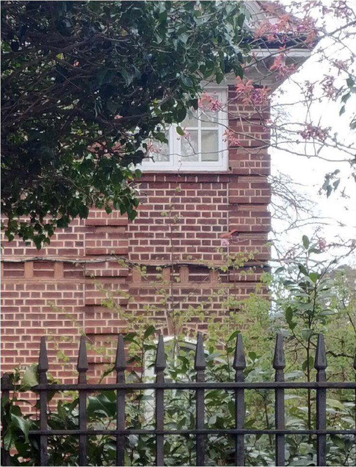
Brick quoins express the corner of number 70 Maresfield Gardens with the appearance of two columns supporting the roof
