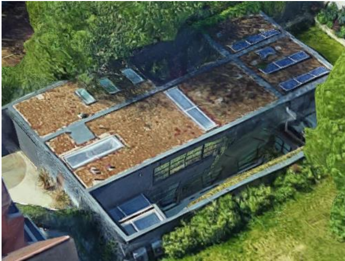
Image 3 - Aerial view of 45a Fitzjohns Avenue
