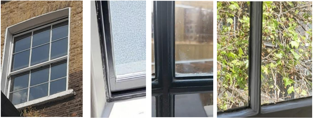
Figure 24. From left: External view of second floor half landing window on the rear elevation above the closet wing; Modern frame of second floor half landing window inside an older architrave; Detail of the glazing bars of the second floor half landing window which is proposed for removal; Glazing bars of a second floor historic window on the front elevation illustrating a much slimmer profile with finer moulding.
