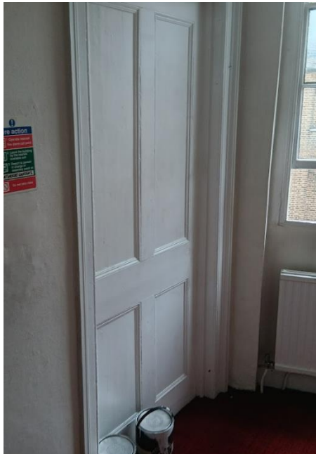
Figure 17. Second floor stairwell of no.63 with historic doorway which would be removed as part of the lift installation for Option 2.
