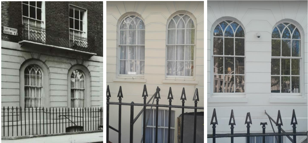
Figure 28. From left: 1965 photograph of the front elevation of The Harlingford Hotel with original tracery windows; Contemporary photographs illustrating the original tracery windows in The Avonmore Hotel (centre) and The George Hotel (right).
