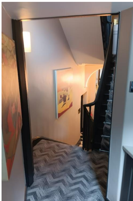
Figure 14. First floor access to closet wing in no.62 and proposed location of lift in Option 1.
