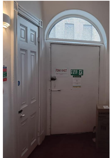
Figure 13. Ground floor main entrance door from Marchant Street and historic doorway on left in no.63 which would provide the lift location for Option 2.
