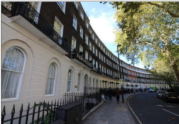
Figure 8. No. 46 – 63 Cartwright Gardens, north Street-facing elevation.
