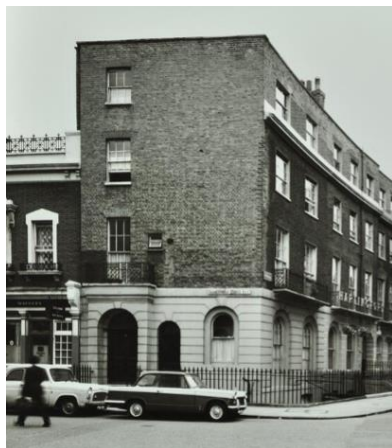
Figure 5. southern and eastern elevation of 63 Cartwright Gardens c.1964
