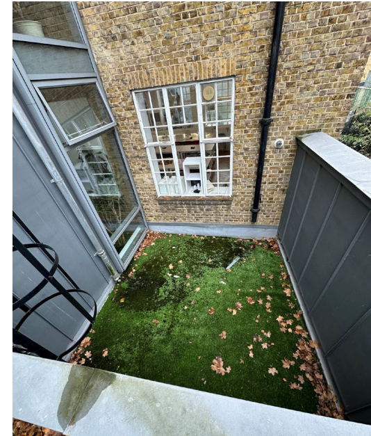
Fig. 5 – Flat Roof where rooflights will be located
