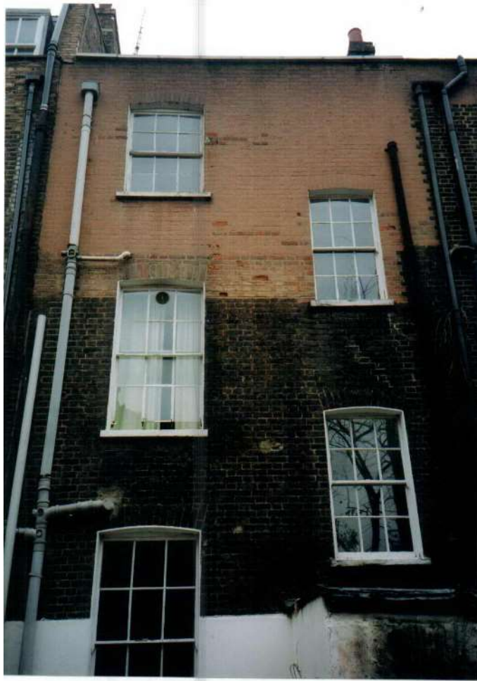
Photograph of rear elevation, showing inappropriate brickwork
