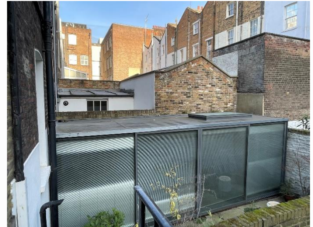
Figure 40 The approved lower ground floor layout at no.15 Thanet Street (left) - planning and listed building consent applications 2006/4473/P and 2006/4474/L. A view looking north showing the highly contemporary extension at no.11 Thanet Street and the structures to the rear of no.12 Thanet Street which fill the depth of the site.
