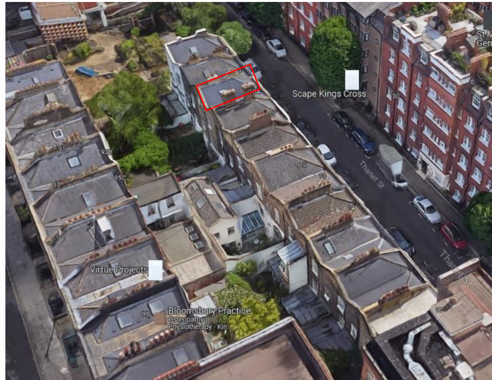
Figure 38 An aerial view of the rear of the listed terrace along Thanet Street showing the variety of form, height and footprint to the rear additions.
