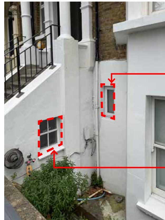
Existing 2no. small windows to west side of front entrance stairs which are proposed to be removed, closed up and finished in matching white painted stucco render
