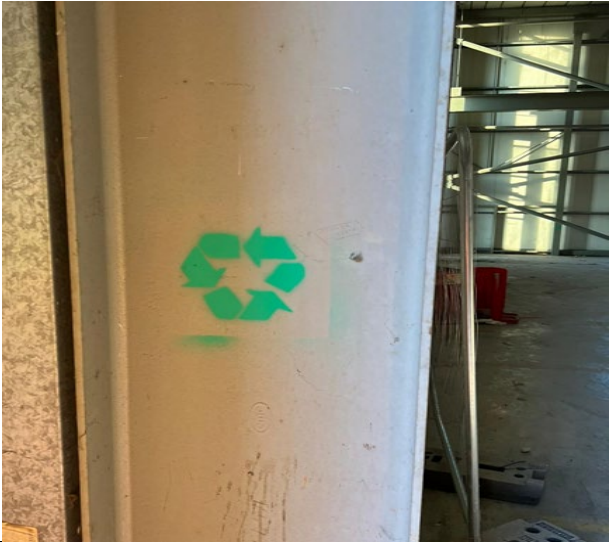
Steels to be re-used are to be marked up on site as shown
