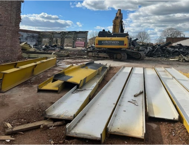
Images of previous cut steel prepared for re-purposing.
