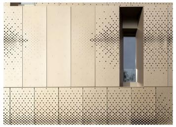
Perforated cladding with simple repeating pattern reducing solar gain:
