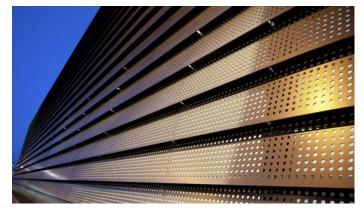
Perforated cladding in bronze with glass and concrete, controlling solar gain and privacy
