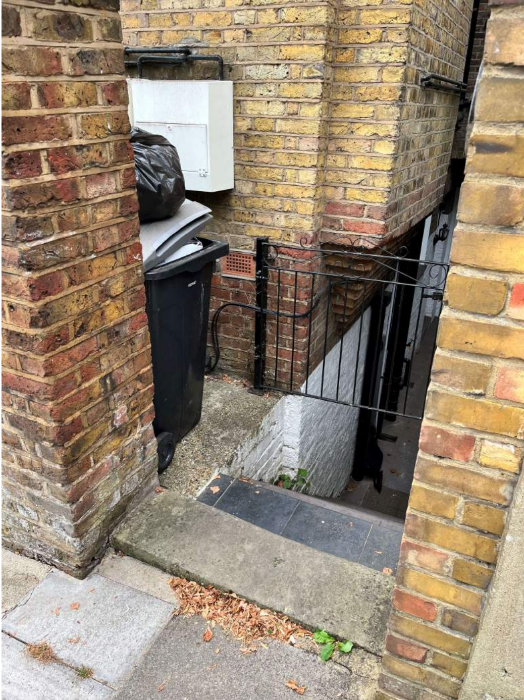
Image 07 – Photograph of the existing side access to the external refuse store of 14 Lyndhurst Road, which requires users to cross over the top of the external staircase to a basement flat without the benefit of a level landing. (July 2022)
