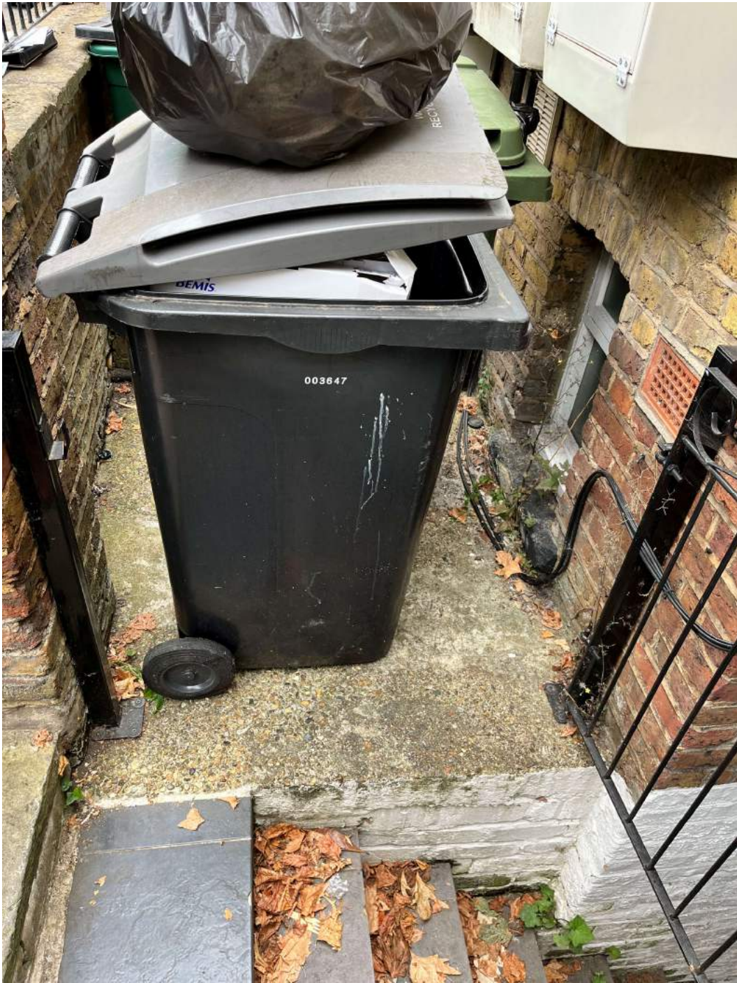
Image 08 – Photograph of the existing side access to the external refuse store of 14 Lyndhurst Road which shows how the users are required to cross over the top 4no. steps of the external staircase to a basement flat in order to empty and access the bins enclosed within. The existing 1.2m wide side access will be in-filled with a 1 metre tall single leaf brickwork wall in matching fair faced brickwork with stone coping atop. (July 2022)
