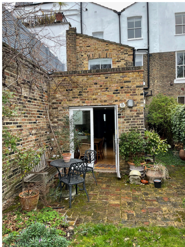
30 Falkland Road - Rear Elevation
