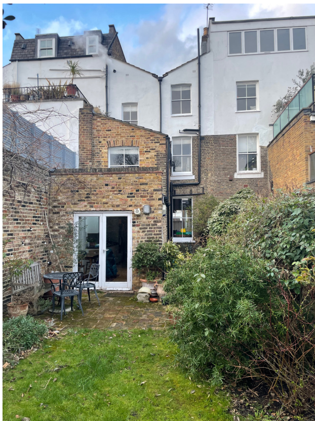
30 Falkland Road - Rear Elevation
