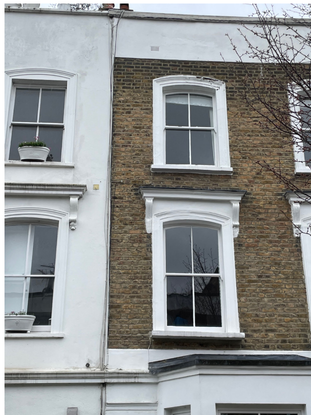
30 Falkland Road - Front Elevation
