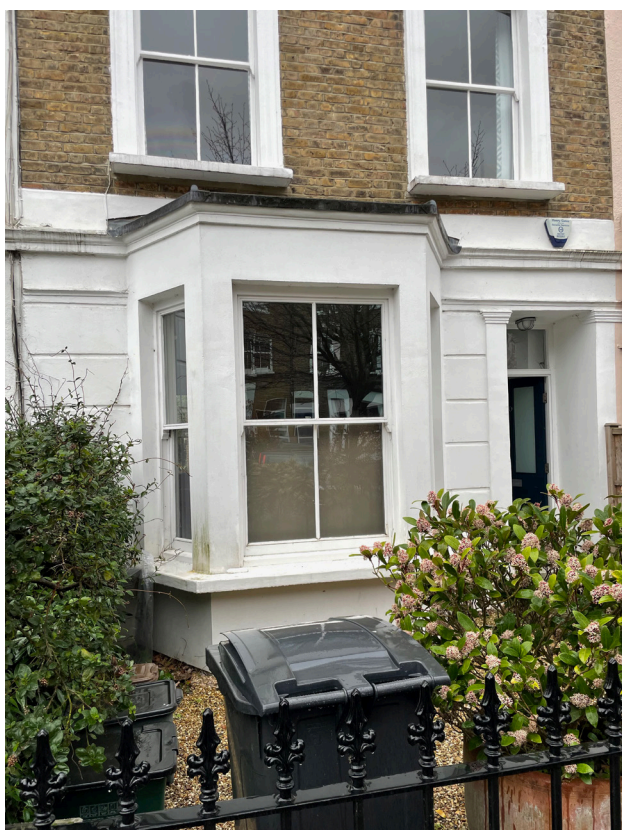
30 Falkland Road - Front Elevation
