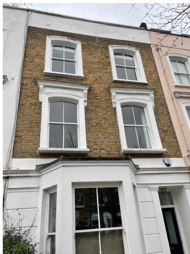
30 Falkland Road - Front Elevation
