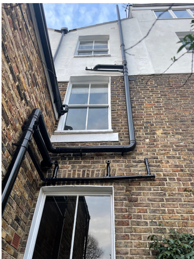
30 Falkland Road - Rear Elevation
