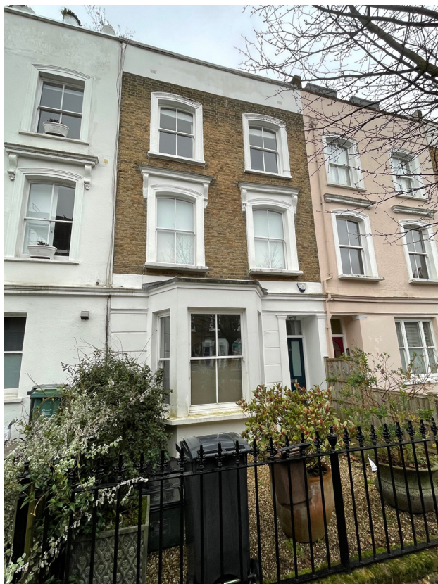
30 Falkland Road - Front Elevation
