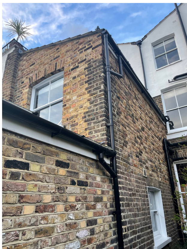
30 Falkland Road - Rear Elevation
