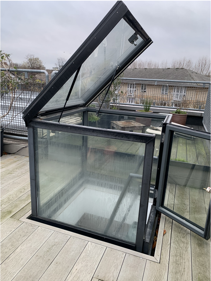
PH.2 Existing non original glass box rooflight - external view
