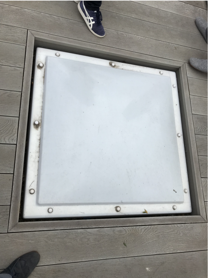
PH.3 Existing polycarbonate domed rooflight
