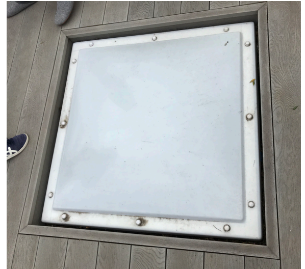
Existing domed polycarbonate rooflight
