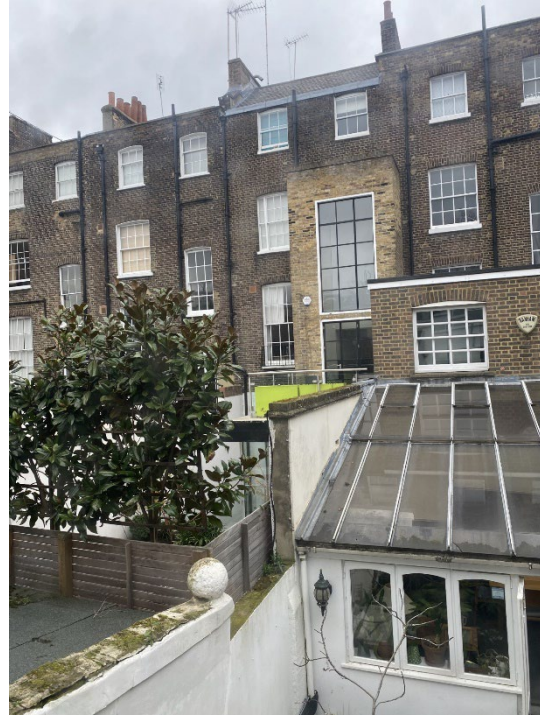
Photograph 2 – Rear elevation (site to right)
