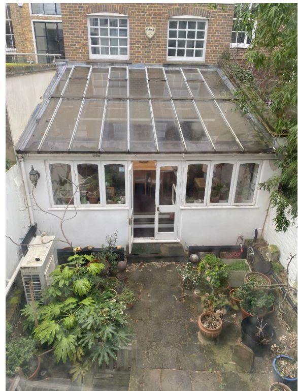
Photograph 5 – Conservatory – Showing boundary walls
