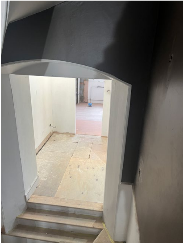
3.15 Opening from staircase onto F1
