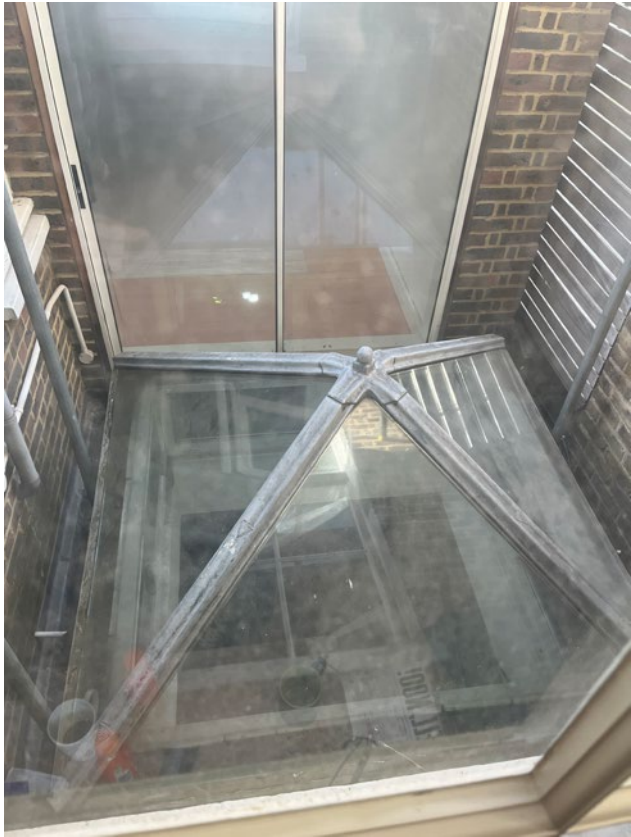
3.25 Pitched rooflight in first floor lightwell
