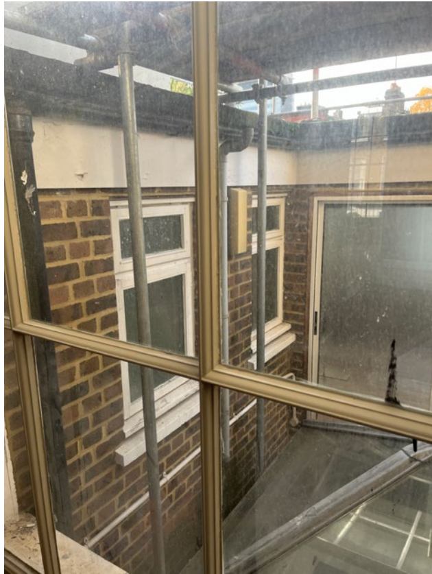
3.26 View south onto first floor lightwell
