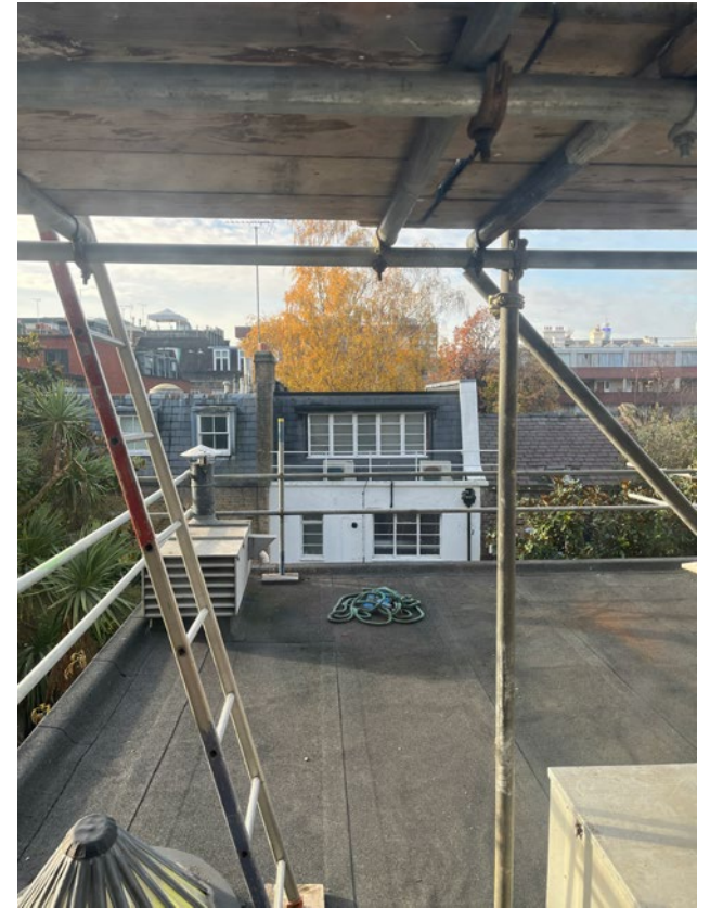
3.24 Flat roof of rear extension showing extract and first floor skylight
