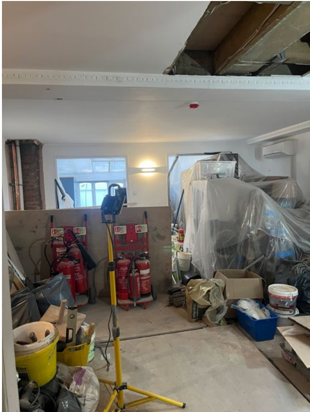
3.9 View west in G1 towards conservatory
