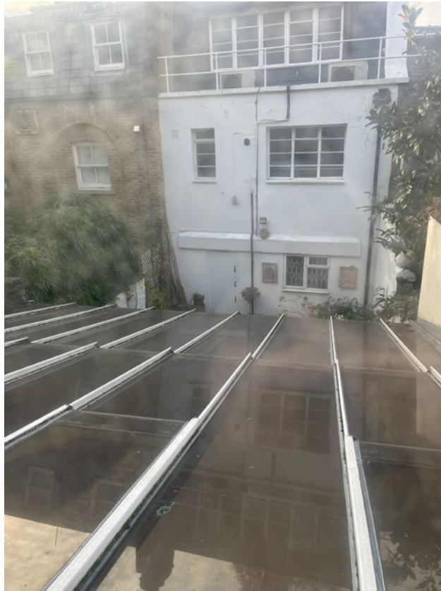
3.23 Glazed roof to conservatory as seen from first floor
