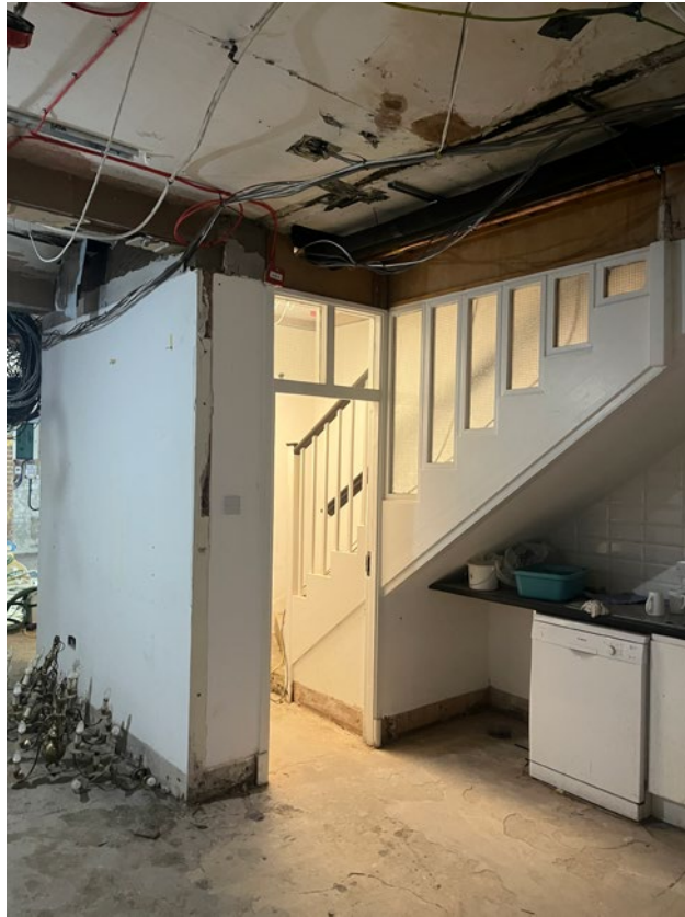
3.3 B1 showing modern doorway and overhead
