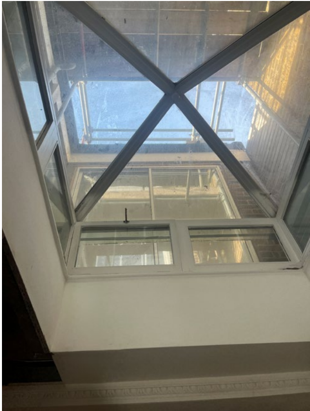
3.12 Skylight in G1
