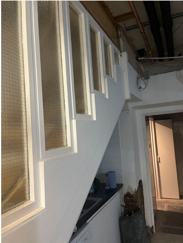
3.2 Wire-glazing in place of balustrade
