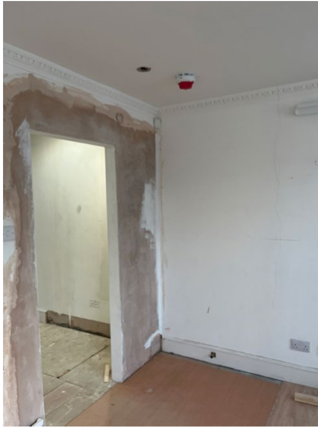
3.19 F2 looking east towards F1
