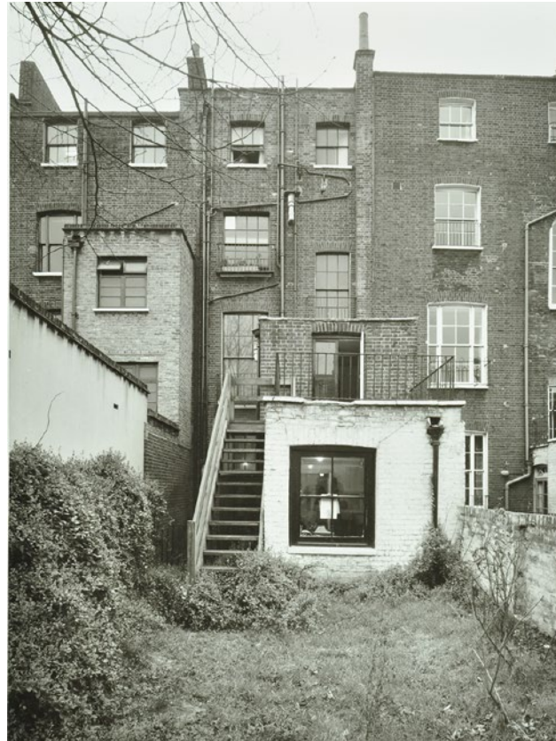
2.13 Rear elevation of 25 John Street, 1975 (London Metropolitan Archives)
