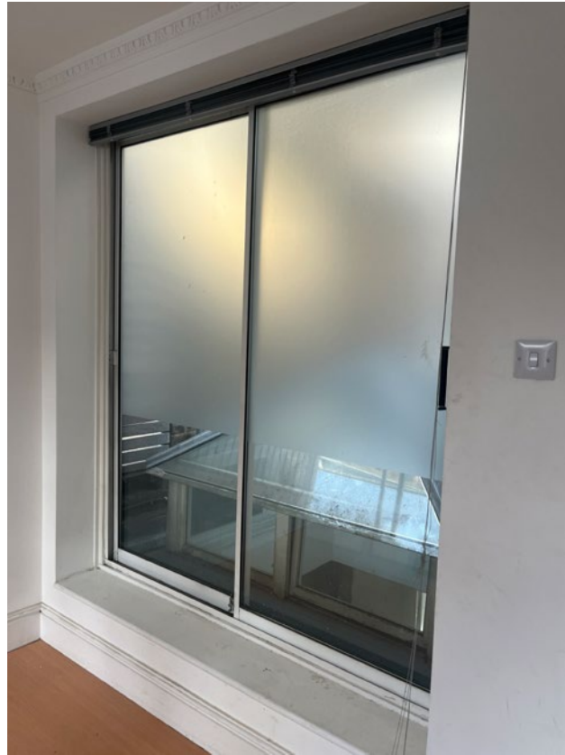
3.21 Sliding door onto lightwell
