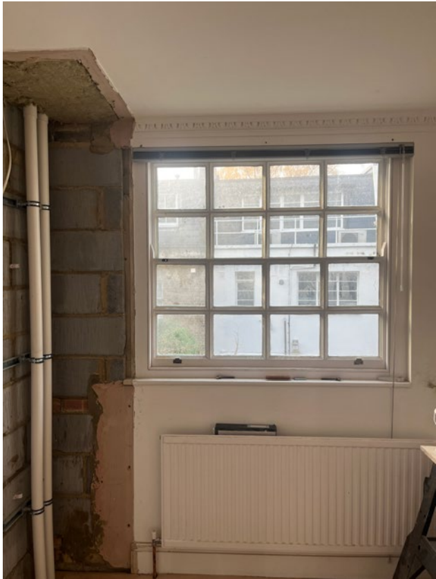
3.20 Modern sash windows to west wall of F2
