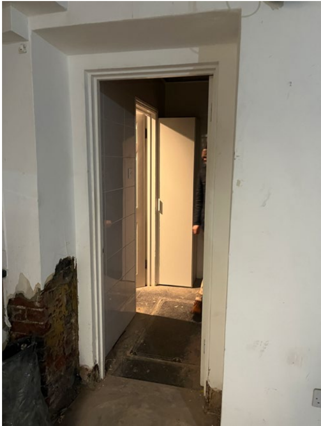
3.5 Doorway from B1 into B3
