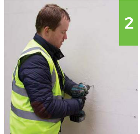
Drill the holes
