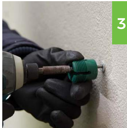
Plug & screw the fixing
