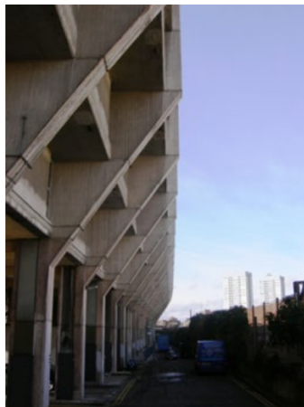
Photo of the existing concrete fins from report
