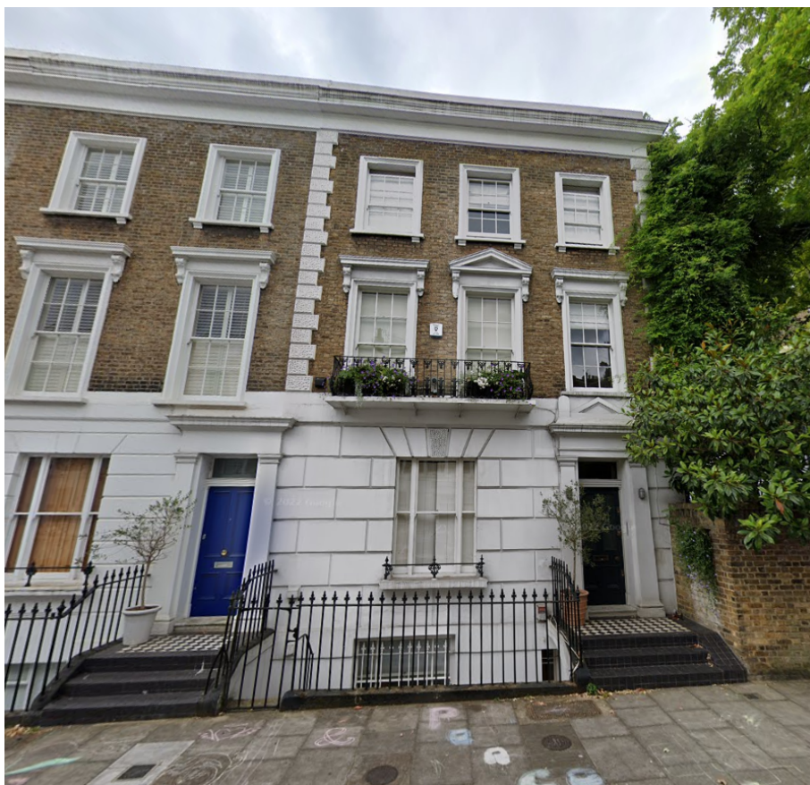
Front of 1 Rothwell Street
