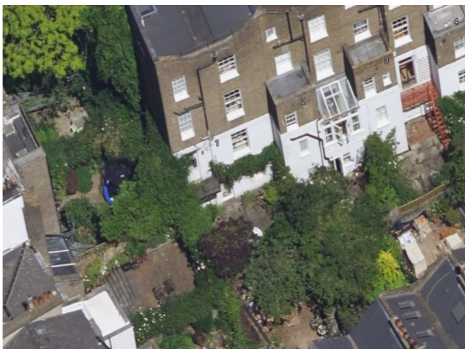
Aerial view of rear of 1 Rothwell Street
