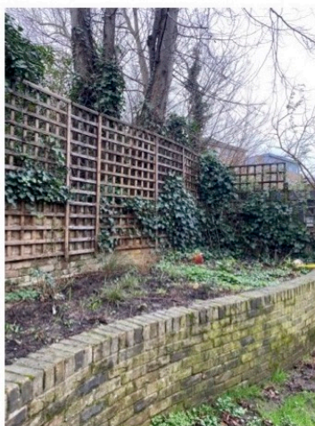
Initial main stem of tree T1 and retainers viewed to south
