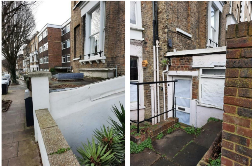
The infill between the house and pavement
