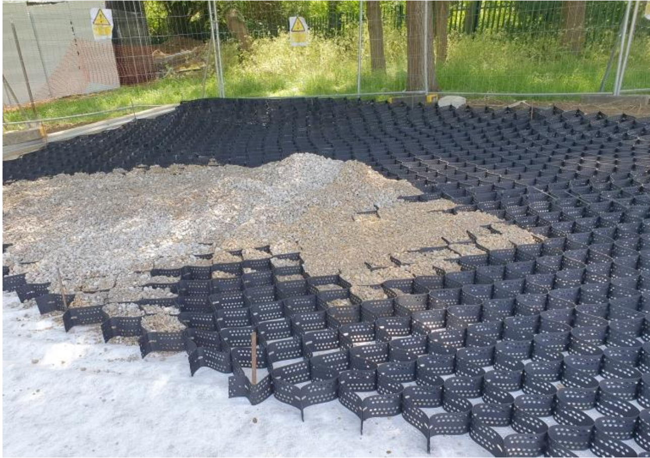
Fig 5: EXAMPLE OF INSTALLATION OF CELLULAR CONFINEMENT SYSTEM
