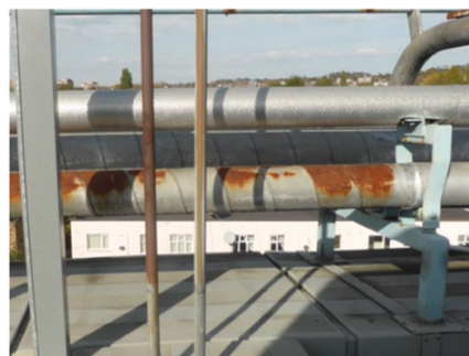
Roof mount located on Block A roof
