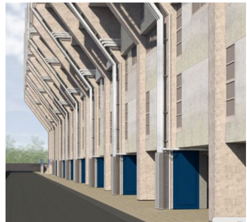
Photo of concrete fins with the new proposed pipework from the report.
