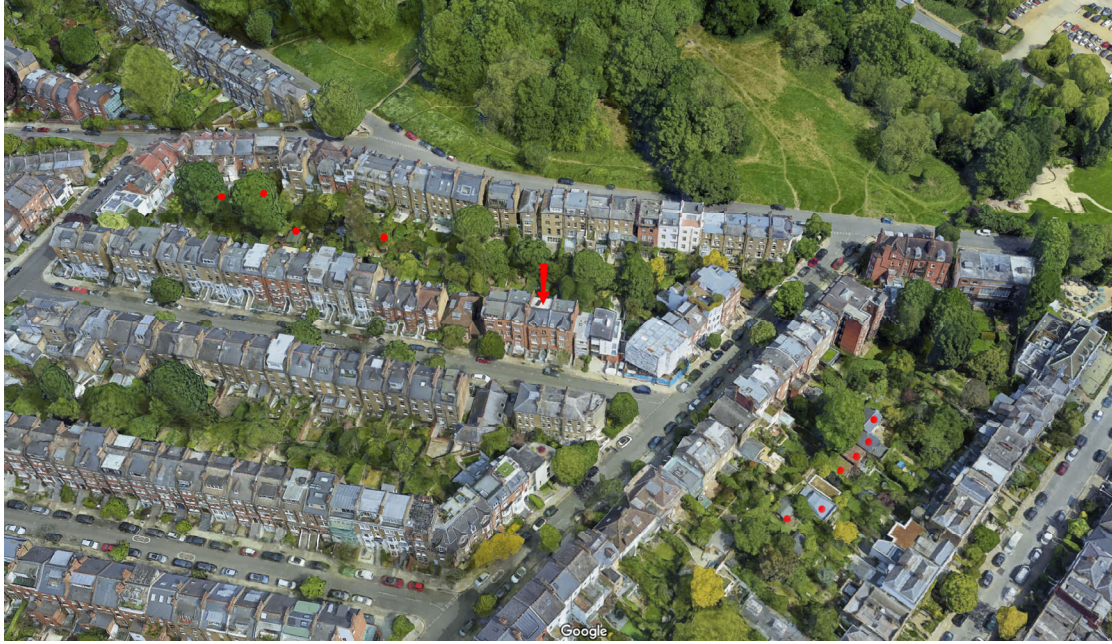
Garden Rooms/sheds are shown with red dots. The arrow shows 43 Denning Road Diagram 1
