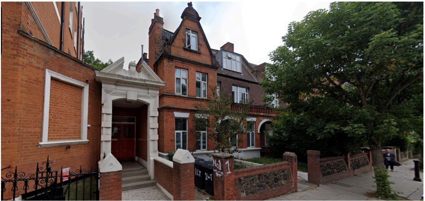
Number 1 Lymington Road at the centre of the image showing the side alleyway with access to the rear garden and proposal site visible between the subject property and the impressive entrance door to the neighbouring Lymington Mansions. The house is located close to West End Lane in the heart of West Hampstead.
