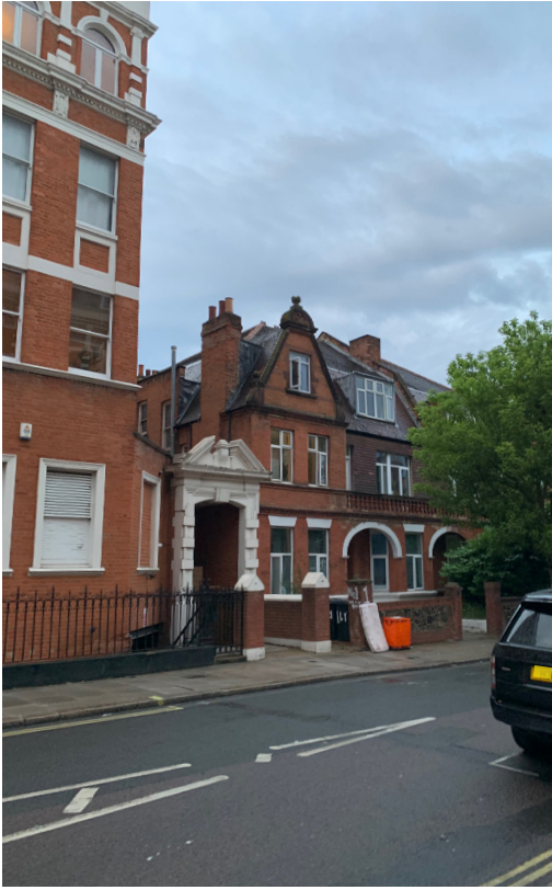
View to the front elevation to number 1 Lyminster Road.
