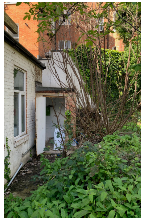
Views to the existing rear extension and garden.
