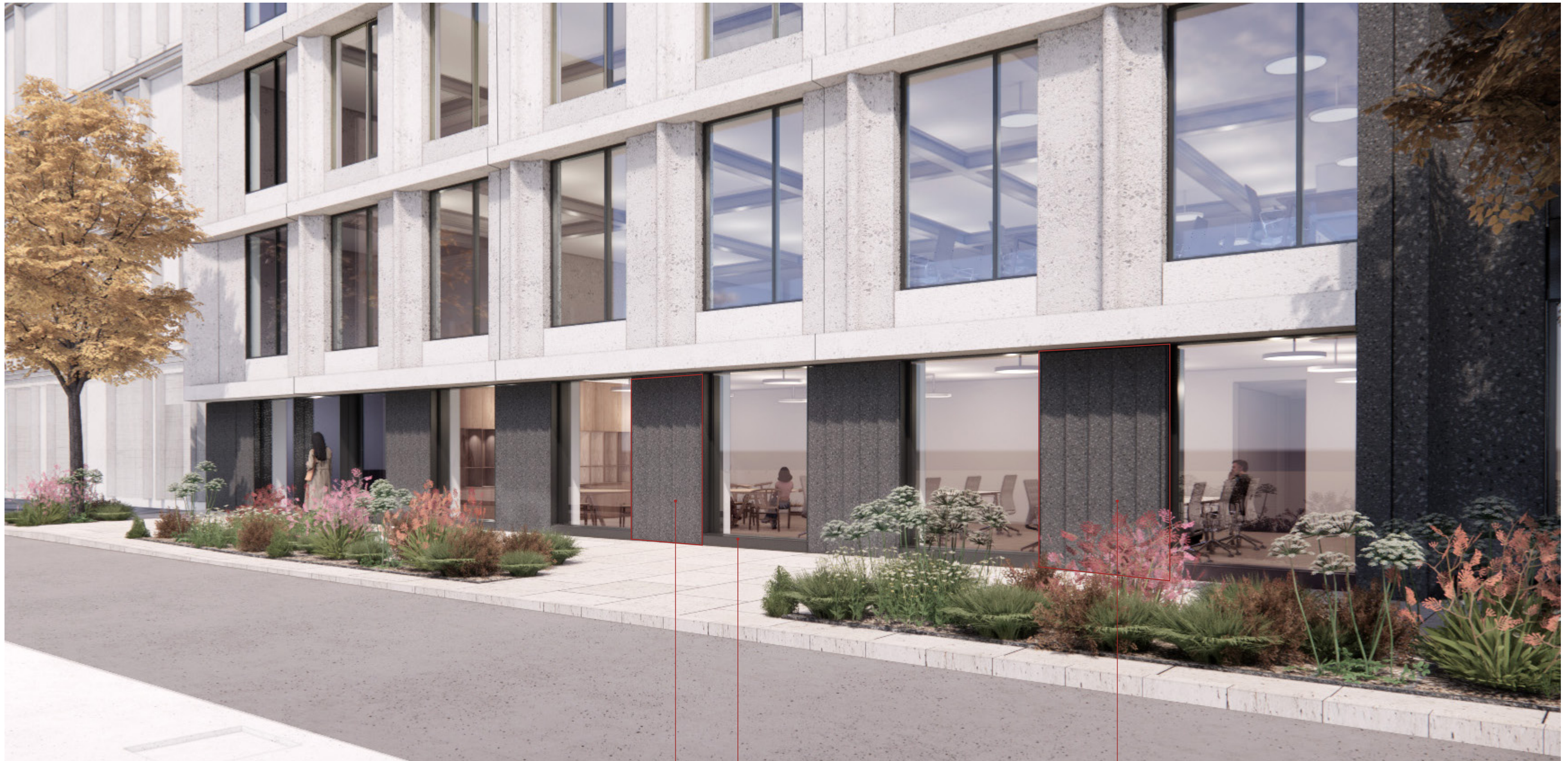
Whitfield street Ground Floor Frontage - Precast panels
