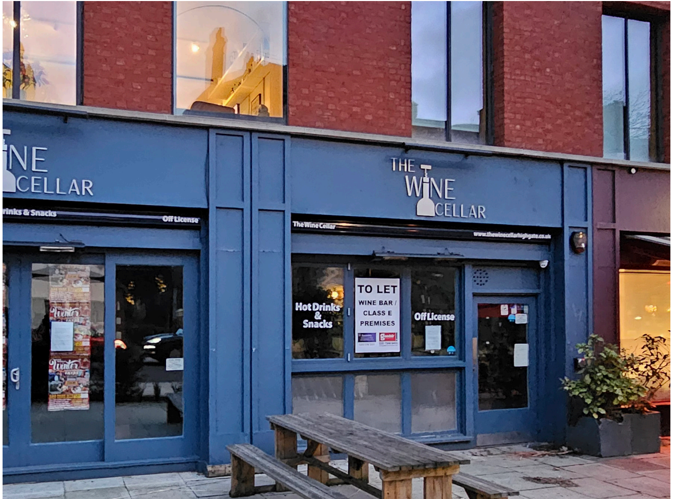
Photo 4 - Main entrance close-up, with ventilation intake grille dropping lower than the shopfront, above the main doors
