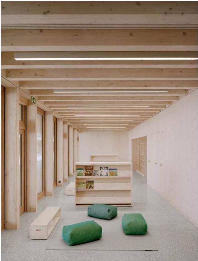
Exposed timber frame with glazed infills
