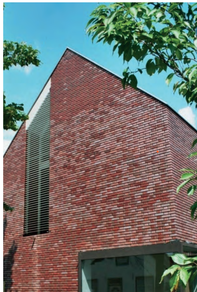
Louvred opening within brickwork
