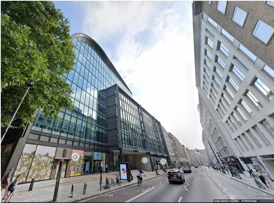
Image 1: Mid City Place and High Holborn (A40), facing west.
