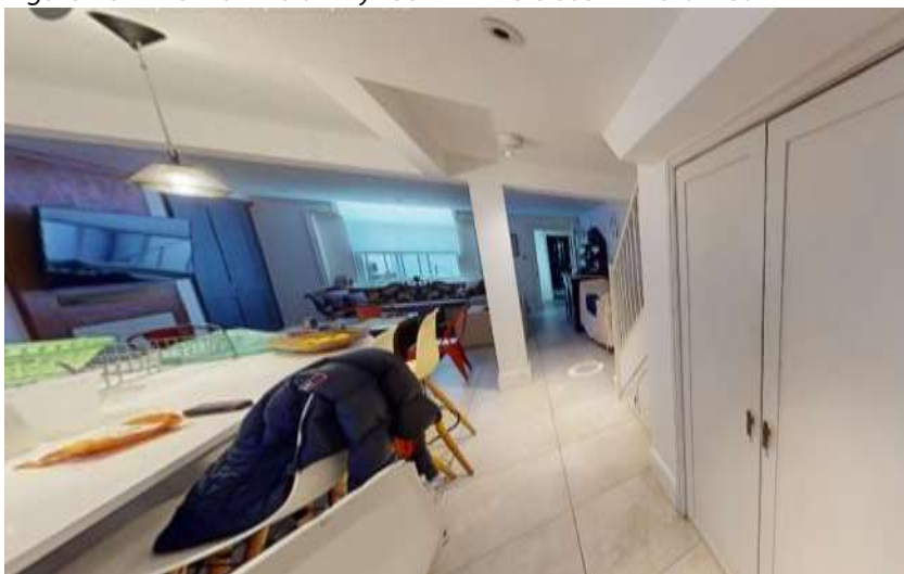
Figure 17 – View of the kitchen and living room area. The wall between front and rear room removed with downstand beam and single column retained. Chimney breast are retained, but no fireplace/stove remains. No cornices.
