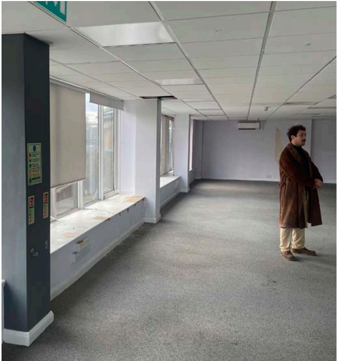
Some floors have very limited floor to ceiling height which compromises future fit-out and MEP.
