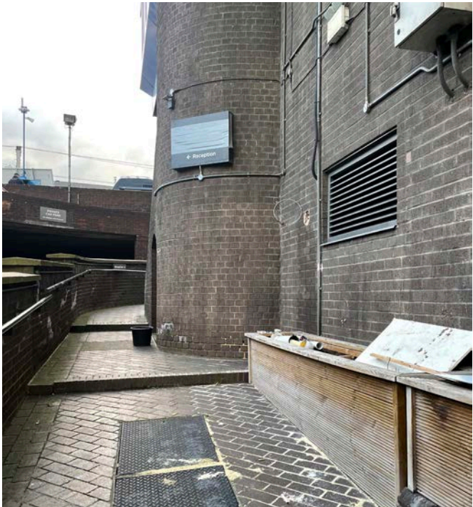
Inaccessible stepped ramp towards reception space. Entrance is set approximately 2m above CFR.
