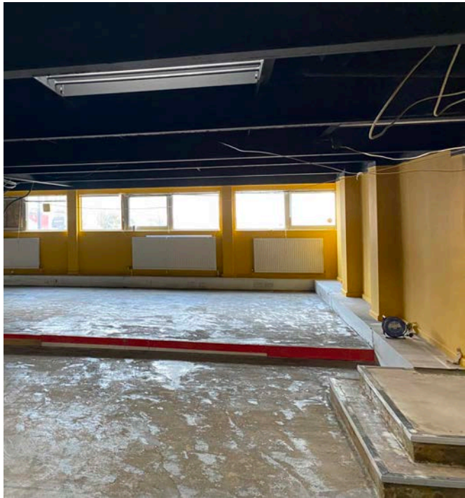
Varied slab and floor finish levels within each individual building or room.
