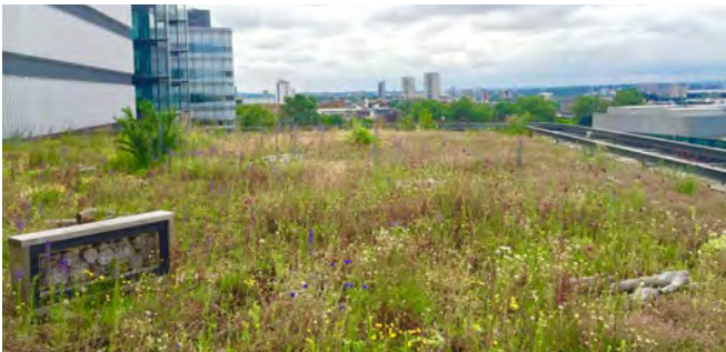
Biodiverse green roof area with invertebrates habitat features
