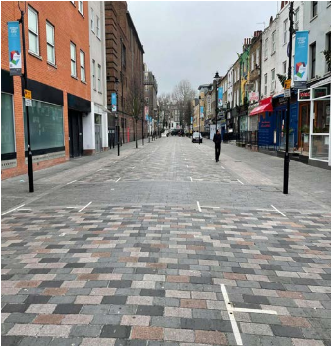
Locally at Inverness Street market new stone setts provide accessible surface finish with similar historic of cobbles
