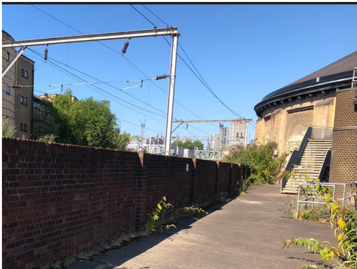
Figure 10 - Existing steel escape staircase.
