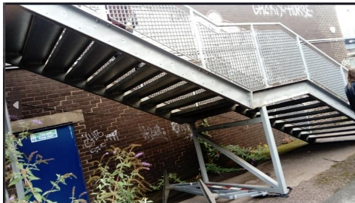
Figure 12 - Existing steel escape staircase.
