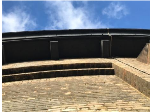
Photo 8: Gaps within the soffit of The Roundhouse
