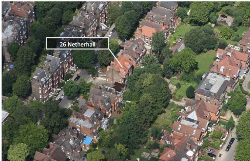
Figure 2. Aerial View of Site looking North
