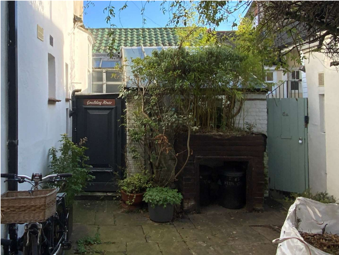
Rear elevation with entrance gate (left), white-painted brick wall with planter in front and modern glazed roof over. The window adjacent to the gate serves the ground floor WC. The gate to the right is the entrance to the adjacent property.
