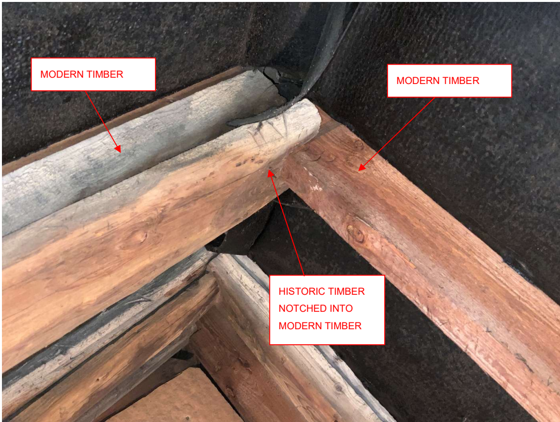
Historic timber notched into modern timber roof construction
