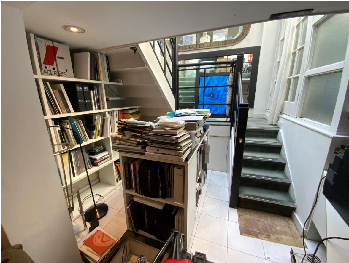
Ground floor rear stair enclosure facing west
