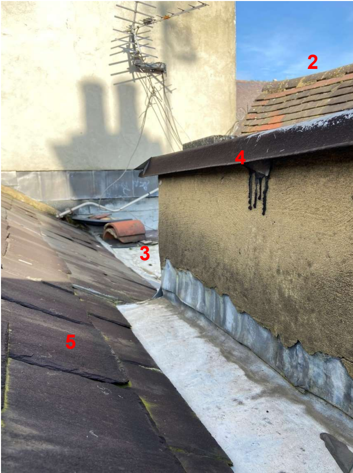
View through rooflight showing elements 2,3,4 & 5
