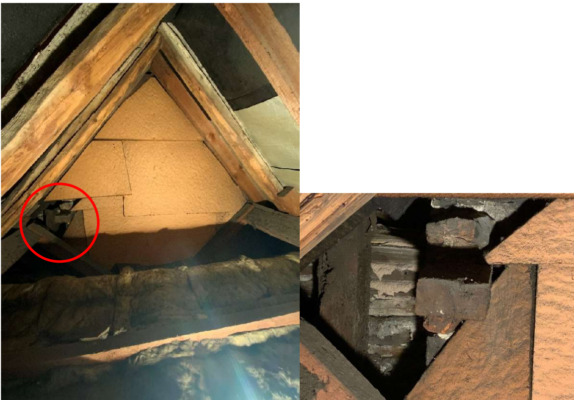
North gable with fibreboard covering; behind there are vertical timber studs with timber laths with a rendered finish The remains of a purlin is also visible, which has been cut through (right).
