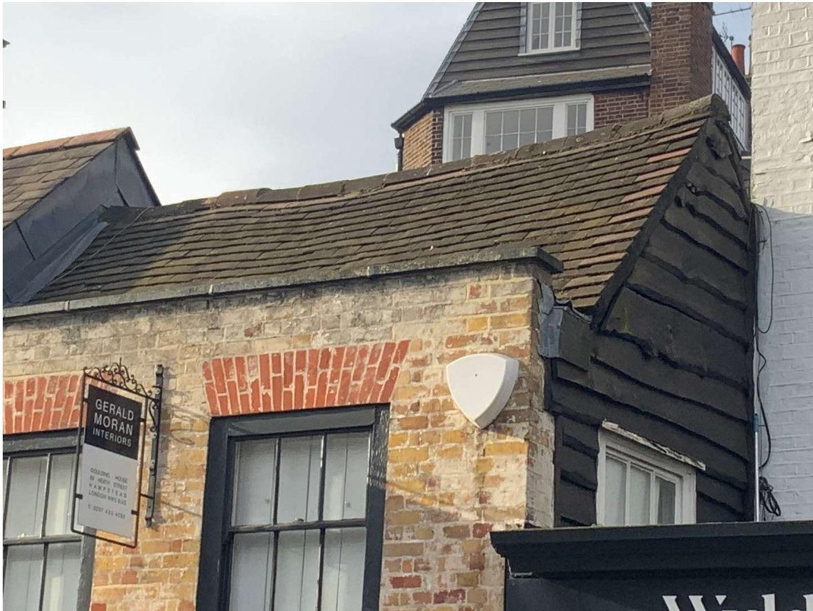
North elevation with weatherboarding and concrete tiled roof.
