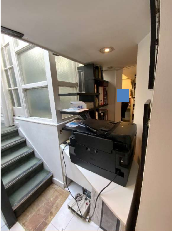
Ground floor rear stair enclosure facing north-west
