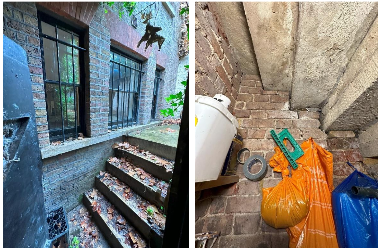
Figures 14 & 15: An external view of the affected windows at lower ground floor level (left) and a view of the underside of the external garden steps from upper ground floor level, showing their full concrete construction (right).
