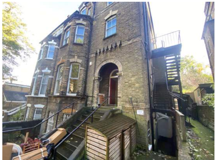
Side view no. 27 Thurlow Road
