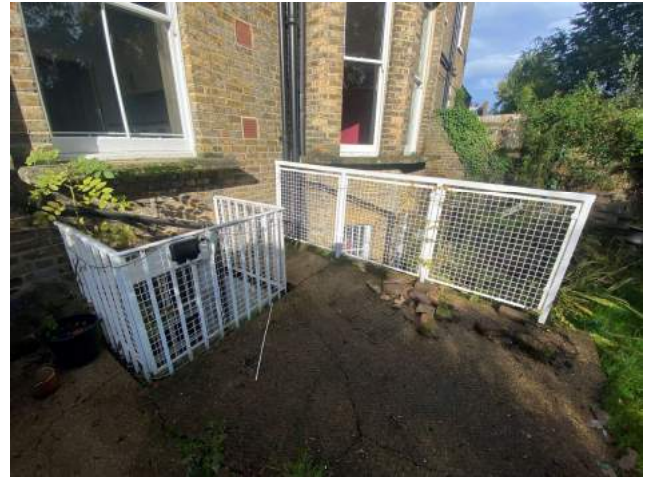
Rear lightwells with metal railing
