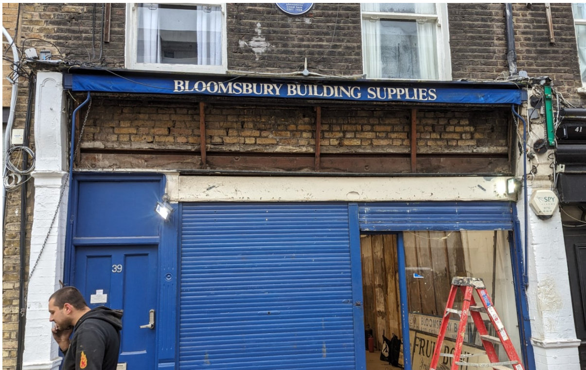
Figure 16: Exposed beam above shopfront opening,
