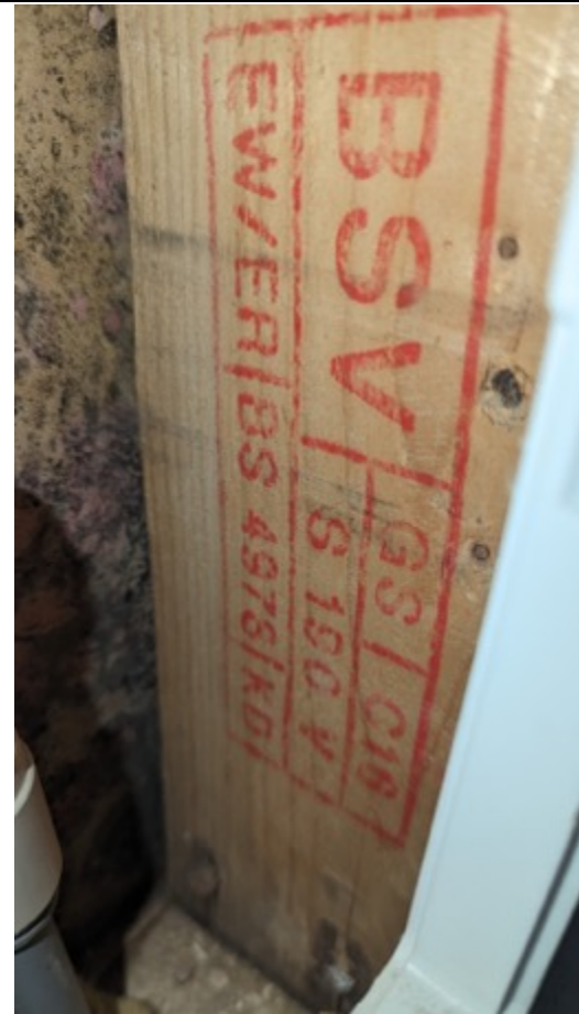
Photo 08: Second floor flat showing grade stamped timber stud
