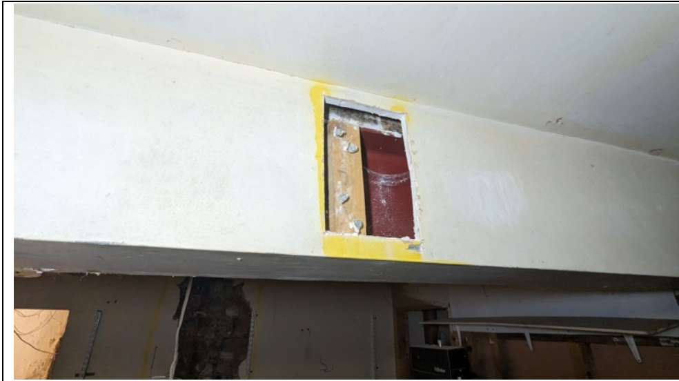
Photo 25: Downstand bulkhead reveals RSJ at high level in basement
