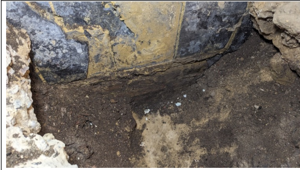
Photo 19: Manhole at rear of basement. Flow direction towards front of building, lateral intercept from adjacent SVP
