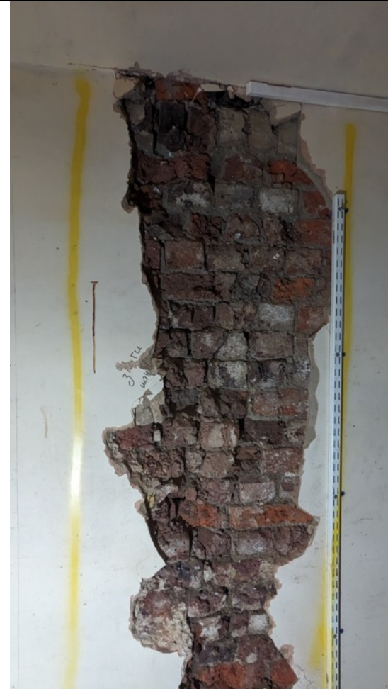
Photo 24: Central spine wall. Cracking has manifested through the brickwork. Damaged bricks, loose and spalling mortar, soft crumbled face to bricks. Repairs / reinstatement required
