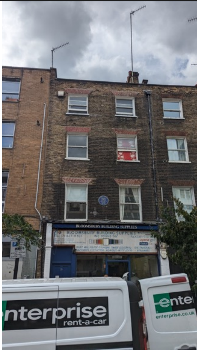
Photo 01: Front elevation taken from street opposite
