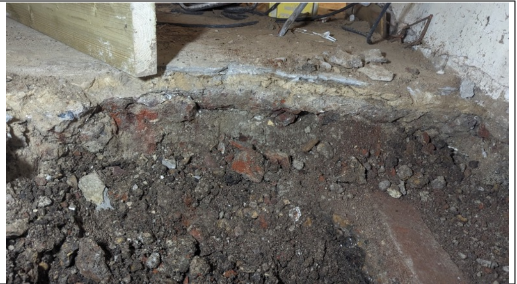
Photo 20: Trial Pit One adjacent to spine wall. Showing thin screed, slab, made ground and projecting concrete footing
