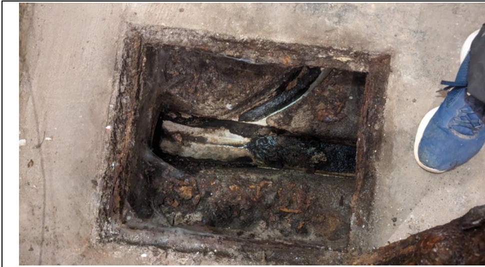
Photo 19: Manhole at rear of basement. Flow direction towards front of building, lateral intercept from adjacent SVP
