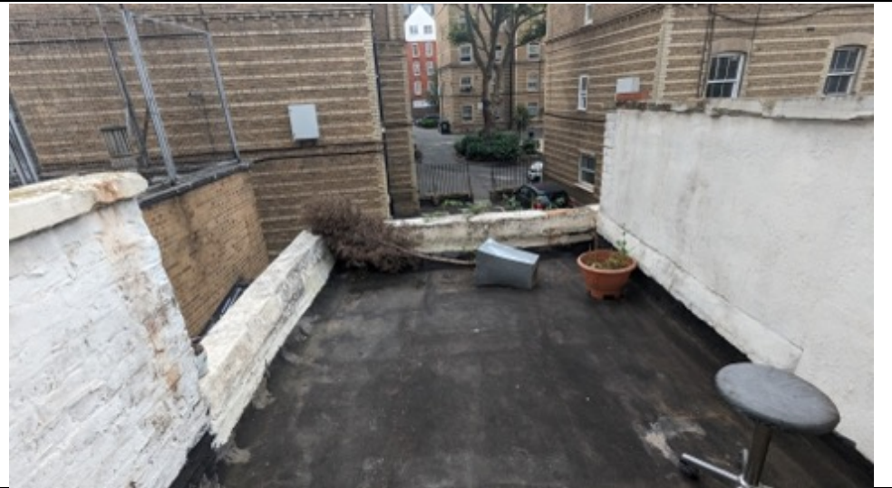
Photo 06: First floor flat roof terrace
