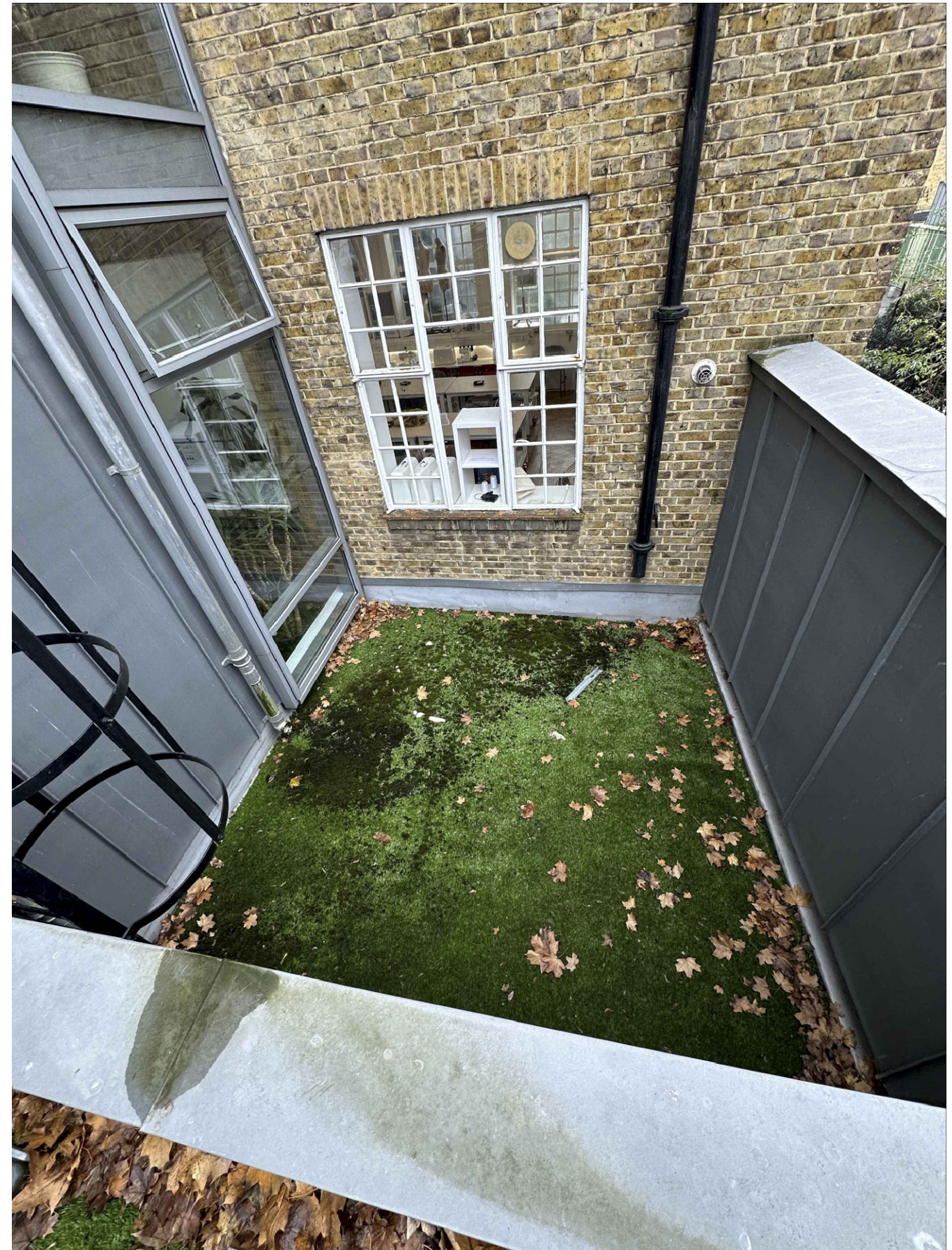
VIEW OF EXISTING FLAT ROOF WHERE PROPOSED ROOFLIGHT WILL BE LOCATED
